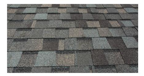
Asphalt roofing or shingle is a type of roofing that uses asphalt material for roof protection and waterproofing. *It is one of the most popular and widely used roofing materials in Utah because it has little up-front costs and is relatively straightforward to install.* The materials used in the manufacture of asphalt roofing include fiberglass and a formerly living organic base.
